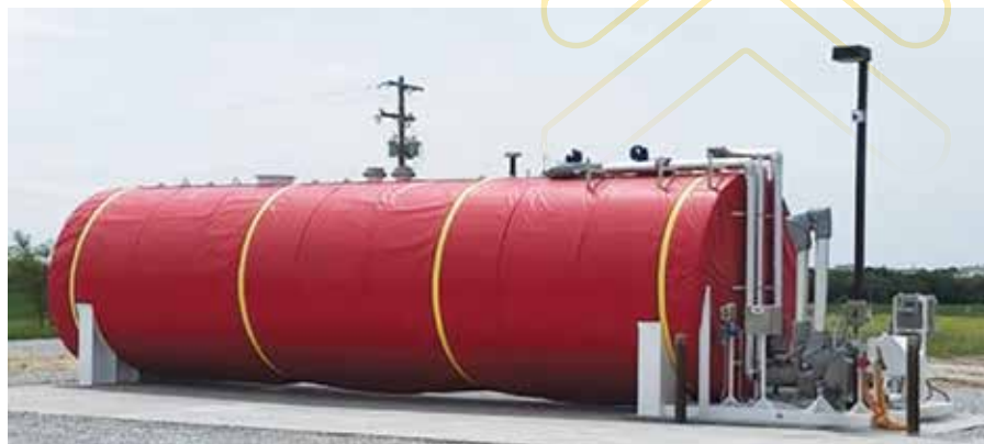
A 20,000-gallon insulated tank with heated arm allows for biodiesel blending in all seasons at the Sapp Bros. site in Geneva.
